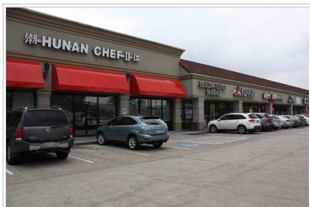
Acquisition of strip mall land at 3809 Southwest Freeway would require moving nine businesses.
